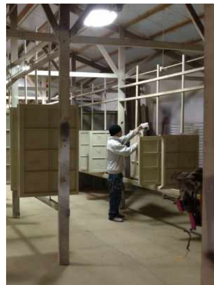
Chosen Windows restoring Straub Hall window sashes in shop
