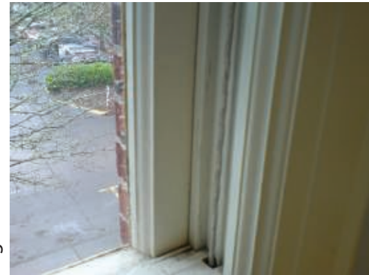
Existing window before treatment
