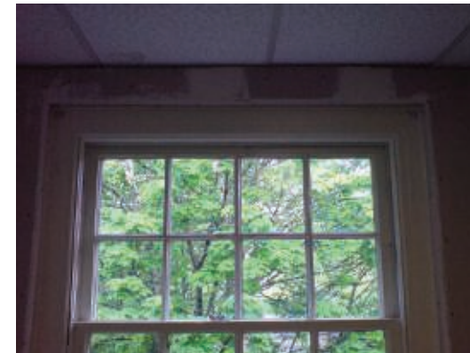
Wall insulation added
