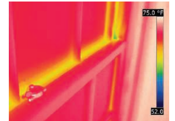
Original sash reinstalled with double glazing replacing original single glazing
