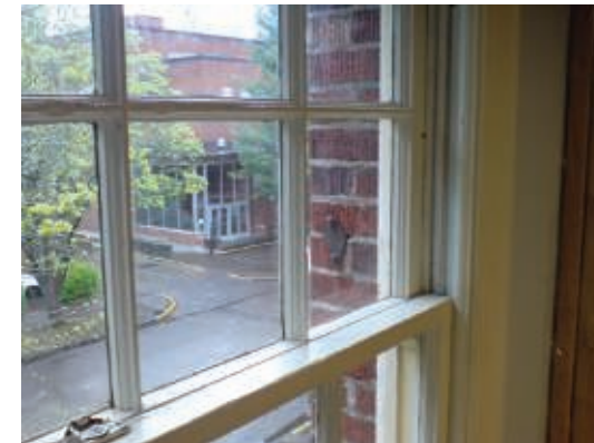
Window has been weather-stripped
