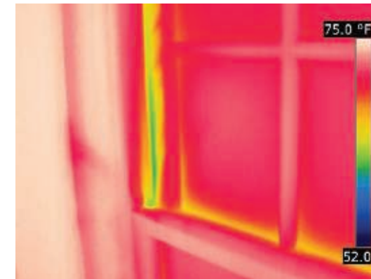
Sash & glazing replaced for units with slip installed
