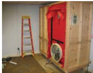
UO Energy Lab testing windows in Straub Hall
